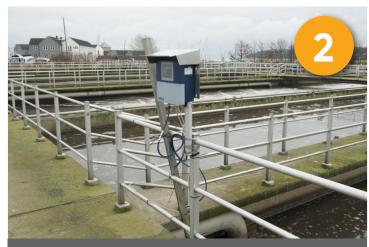
After installing the N<sub>2</sub>O Wastewater Sensor or replacing the sensor head, let the sensor **stabilize overnight**. This will give the best calibration result with zero drift!
