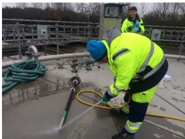
Cleaning of the \text{N}_2\text{O} Wastewater Sensor on top of the reject water tank at VandCenterSyd, Odense, Denmark
