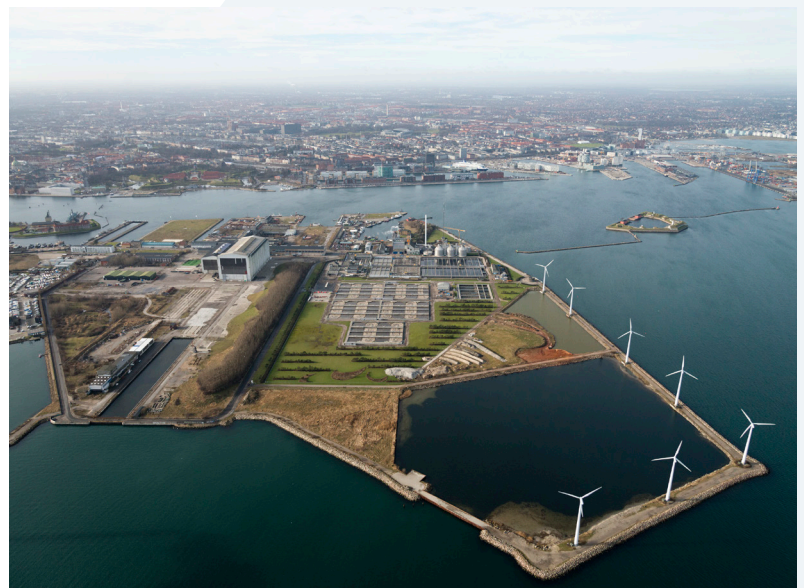
Fig. 1: The 750,000 PE wastewater treatment plant Lynetten, located in the harbour of Copenhagen
