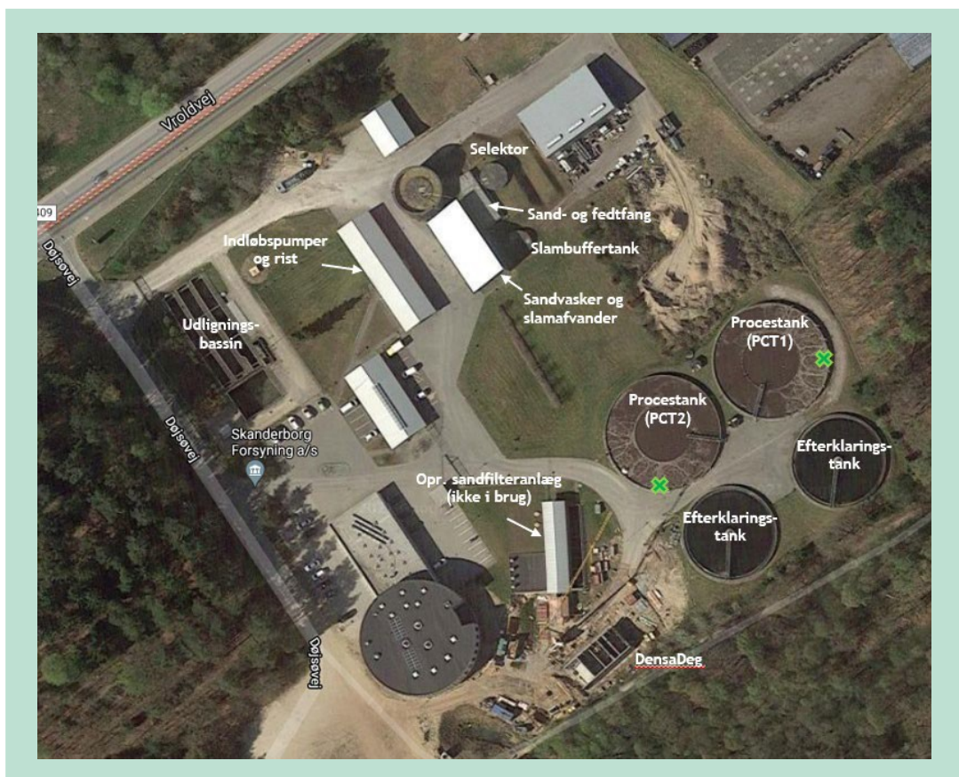
FIGURE Skanderborg1. Central Sewage Treatment Plant. Green cross marks location of nitrous oxide sensor.
