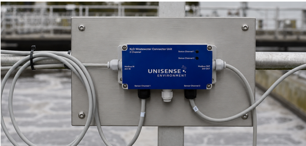
Picture 4: Mounting of an N 2 O Wastewater Connector Unit
